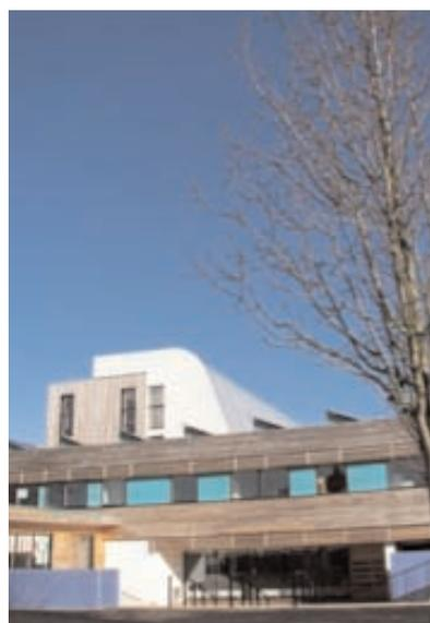
Some financial difficulties led to a process of value engineering, which cut out a number of the sustainable features. For example, motors for the louvres were not included in the final design. They now have to be adjusted by hand, using long poles. Not being able to afford the most suitable glass meant that the atrium is too hot in summer, causing discomfort and costly problems with plaster coming off the walls.
